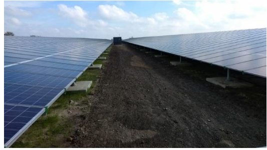
Figure 17 Solar panels placed on stelcon slabs. Source: www.netwerkdurzaamedorpen.nl
