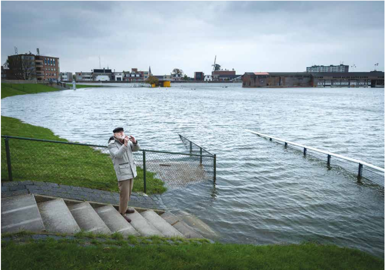
Delfzijl, 22 October 2014: the highest water level measured was 4.06 metres above sea level.
