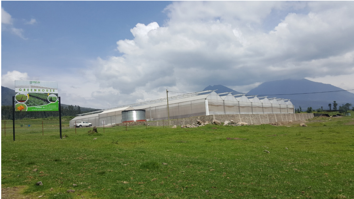
Figure 2.4 Horizon group mechanical and computer controlled greenhouses in Musanze.
