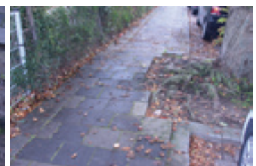
Missing and crooked tiles because of a tree hole.
