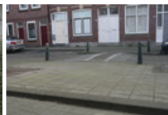
No lowered curb which makes it harder to cross the street at this point.
