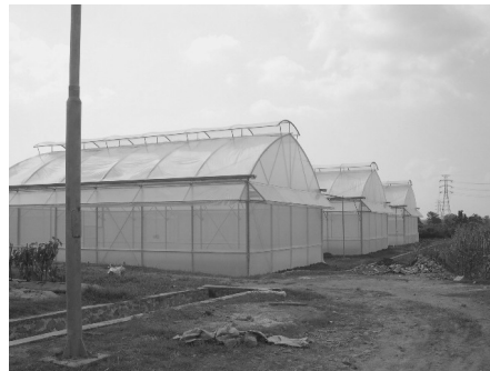
Fig. 3. The new Procult greenhouse design, three greenhouses in a row.
