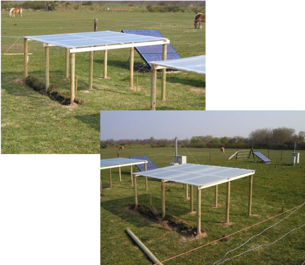
Figure 1 Shelters being built for the dehydration experiment.
