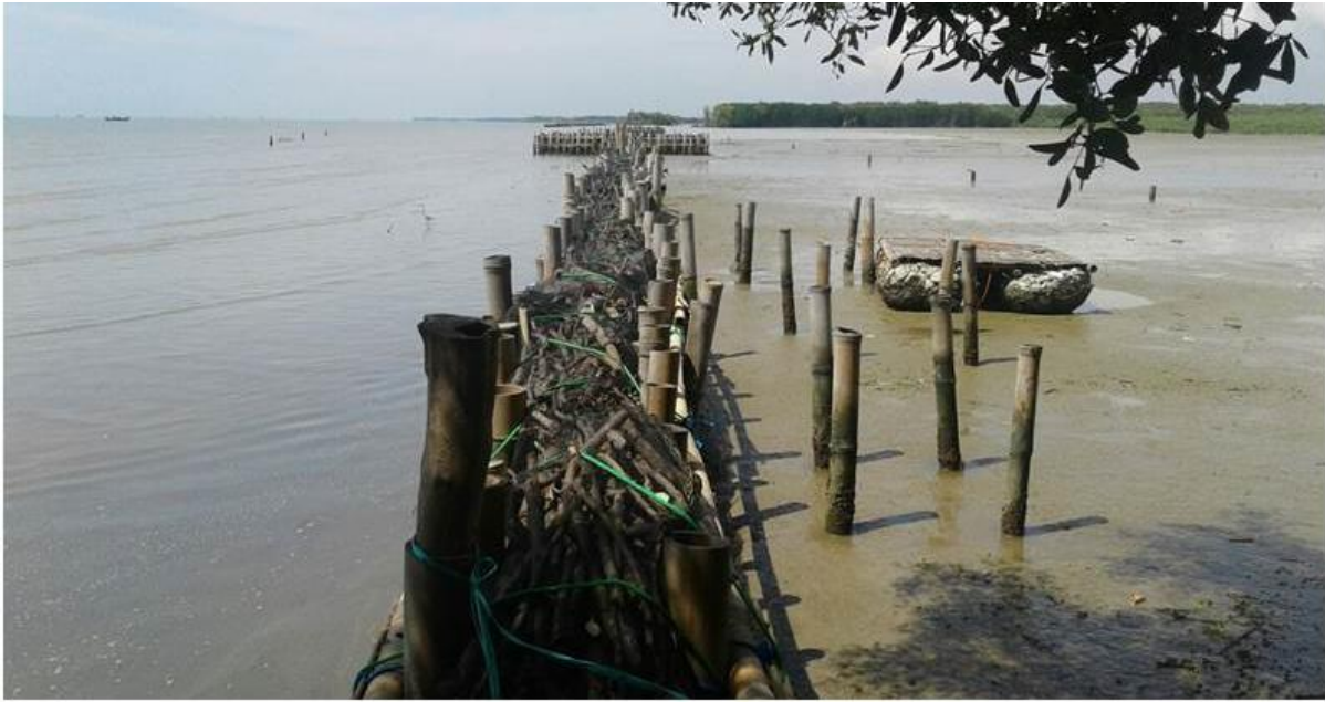
Figure 3. Sedimentation behind permeable dam constructions
