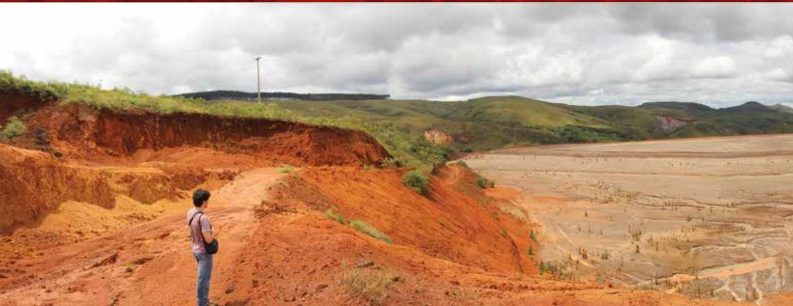
the deserted impoundment area, with the structure of the dam, typically organized in huge staircases made of compacted earth (see Fig. 19). In addition, is possible also to recognize the water collector, where some water of the Company is depurated on the lower part of the landscape and some tailings piles, casually left here and there. Finally, of course, the paths, the drainage system, tubes and pipes are also smaller sign of the anthropic activity on the landscape.
