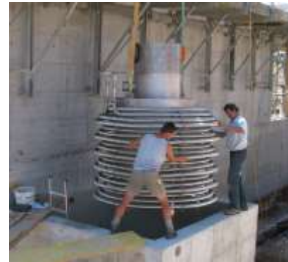
Figure 2. Heat exchanger in a sewer collection pit. Applicable at apartment buildings and flats. (source: www.feka.ch )
