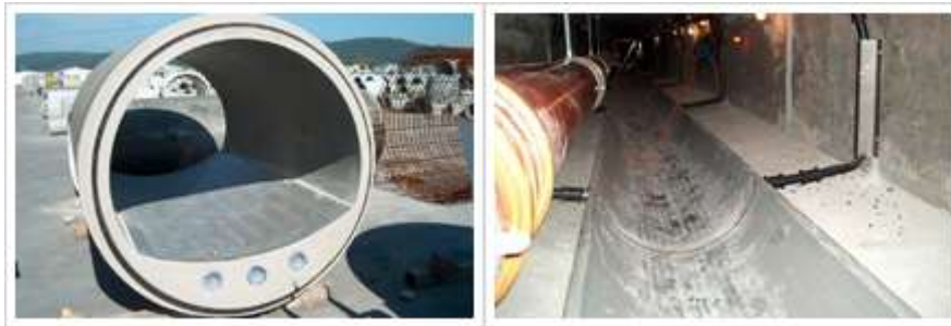
Figure 3. Rabtherm heat exchangers: left integrated system, right: system for implementation in existing sewer mains. (source: www.rabtherm.ch )
