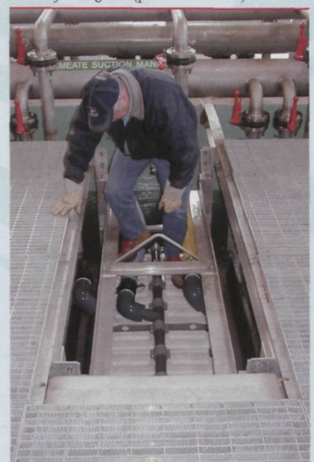
Lifting Zenon membrane section at the drinking water station of Collingwood (photo: DHV Water).
