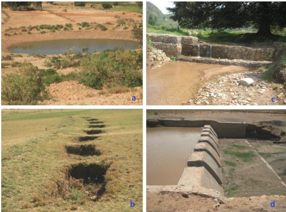
Figure 5.3 Examples of water harvesting techniques implemented in the Gule catchment (a) percolation pond (b) deep trench (c) gabion check dam (d) concrete check-dam pond.
