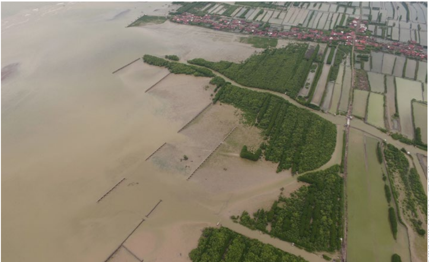
A drone photo of the mangrove restoration project on the north coast of Java near the city of Semarang. The semi-porous dams are visible in the water. They trap sediment, in which mangrove seeds can germinate.
