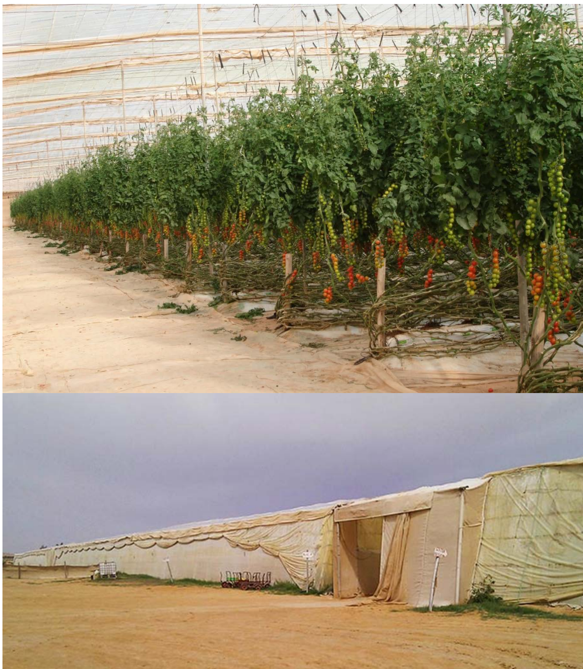
Figure 1 Interior (top) and exterior (bottom) of a Canarian greenhouse, the most common greenhouse in the region of Agadir, a typical size being 1 ha. Air exchange and water discharge is ensured through holes in the roof and by the openings (covered by nets) on the sidewalls. A very limited management of ventilation is done by manually causing splits between adjoining plastic sheets in the roof (top) and lowering/rising the plastic on the sides (below).
