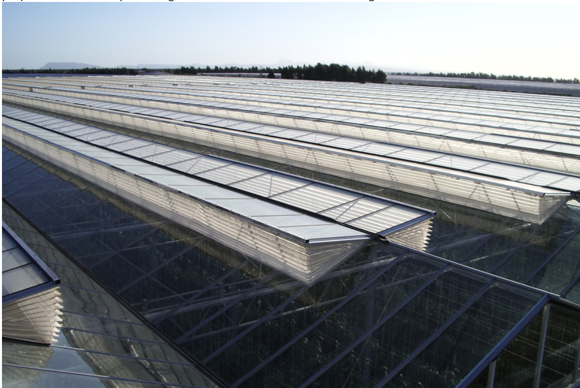
Figure 2 Detail of a Venlo greenhouse with double continuous roof vents implemented with a concertina type anti-insect screen.
