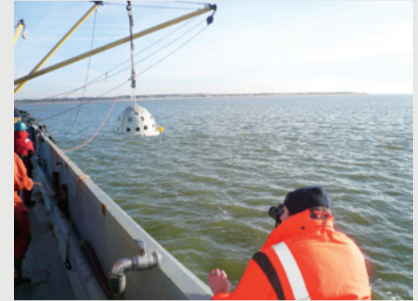
Figure 3: Placing of reef dome at Voordelta location.
