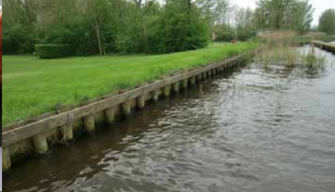
Sheet piling of wooden poles
