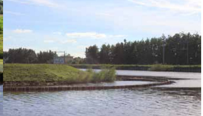
Sheet piling of wooden poles
