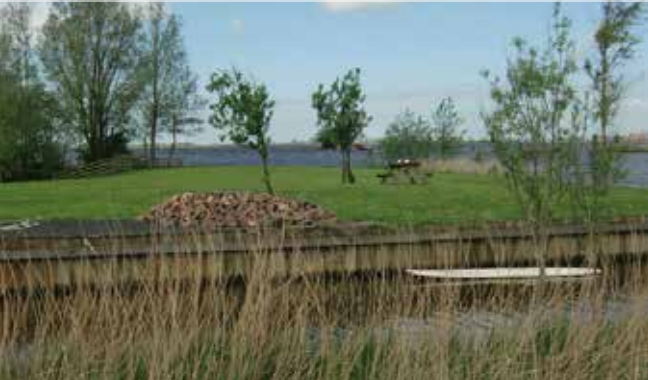
Wooden sheet piling of a couple years old
