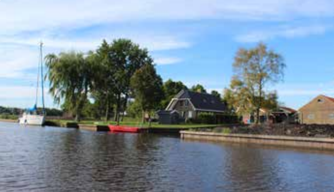
Wooden sheet piling, new
