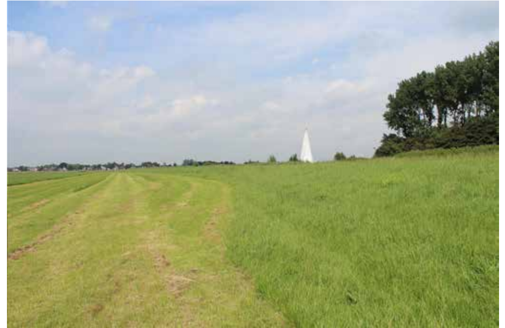
Figure 167 Photo of a regional embankment taken next to the regional embankment
