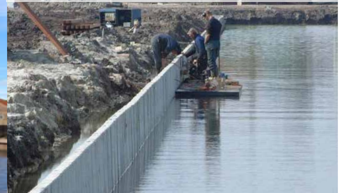
Sheet piling of concrete
