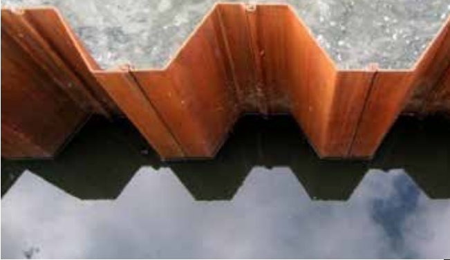
Sheet piling of steel
