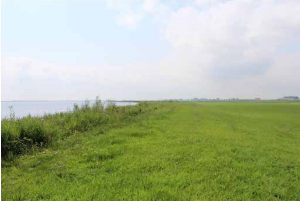
Figure 166 Photo of a regional embankment from the top of the embankment
