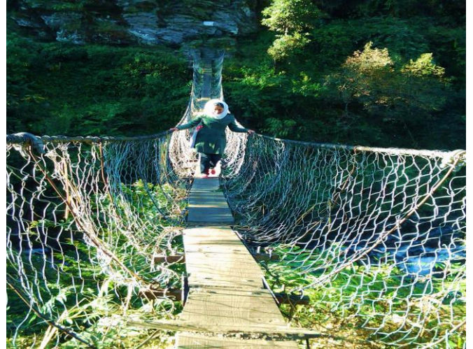
Hanging Bridge over the river
