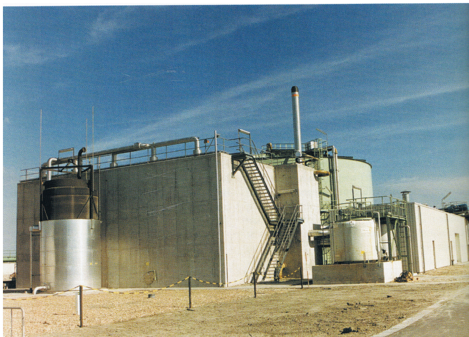
Figure 1.6 Two-phase wastewater treatment plant at Cerestar (Sas van Gent, The Netherlands) (Reith et al., 2003). Methanogenic reactor (UASB) at the front and acidification reactor (CSTR) at the back.
