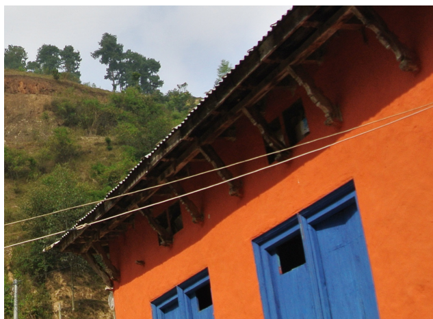
Figure 3.9: Carved wooden struts with overhang of roof
