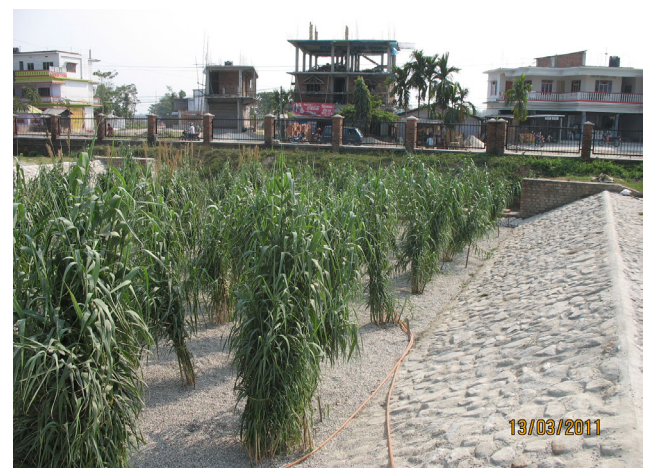
Figure 5.43: Photo of leaching field (P.W.Germeraad, 2011)
