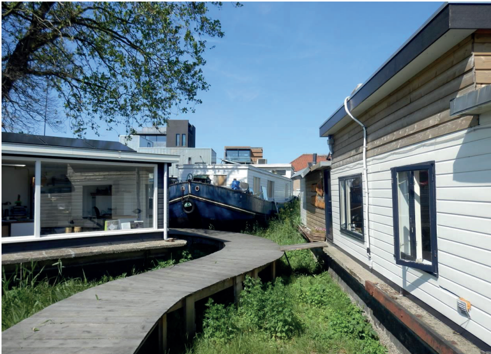
Figure 8. Upycled houseboats at De Ceuvel . Source: The authors
