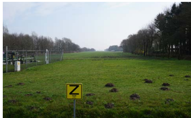
Figure 22: Underground pipeline is visible through a cleared patch of land and signage.
