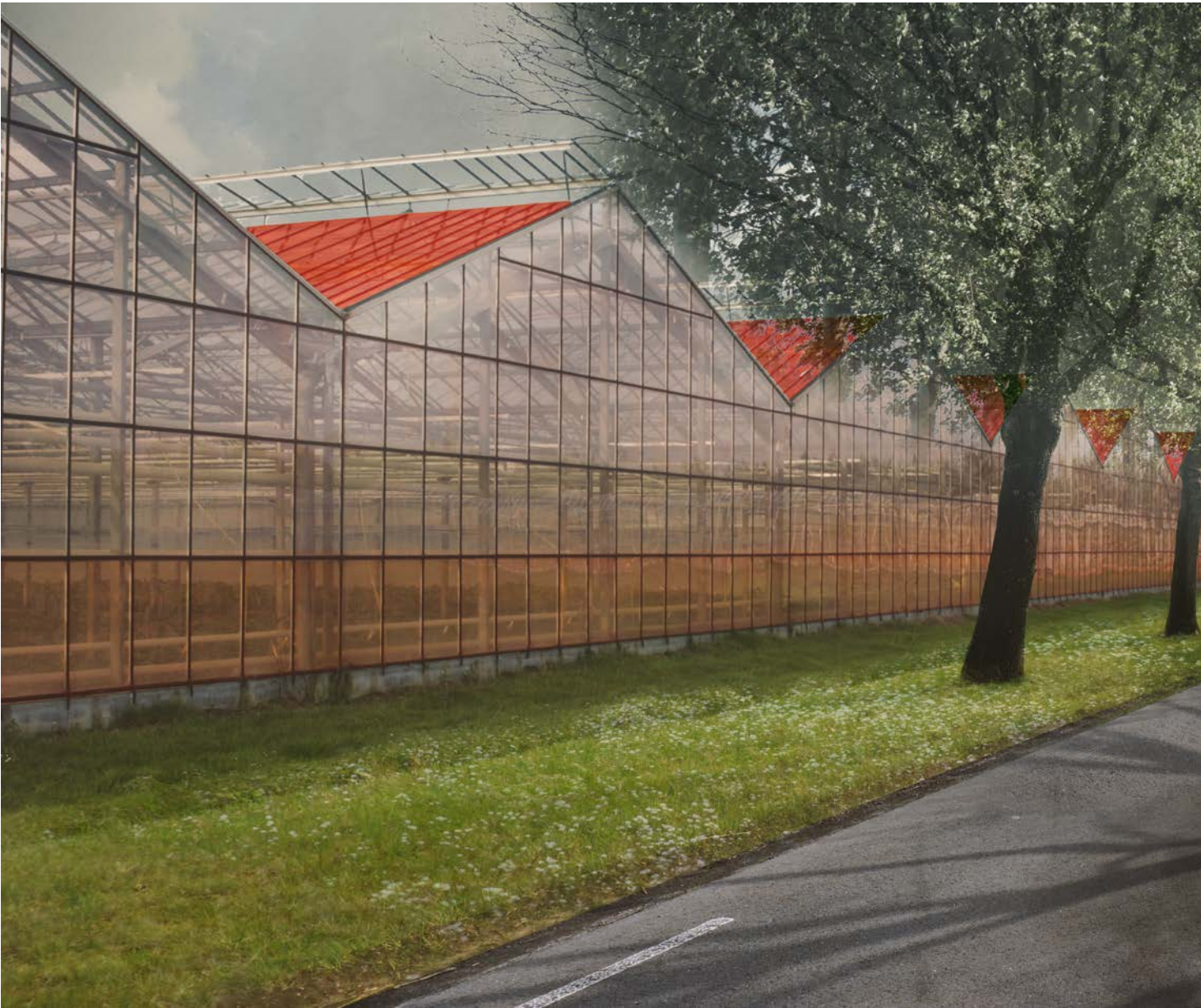
Figure 71: Perspective drawing. Translucent PV panels appear red as they filter parts of the light spectrum not used for photosynthesis. Landscape maintenance on trees and roadside provides biomass.
