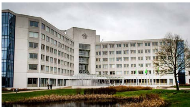
Figure 24: NAM Headquarters in Assen. Photograph by Remko de Waal/ANP.
