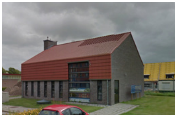
Figure 3.7 Indication of the building type of a Nereda® WWTP (photo retrieved from www.google.nl/maps )
