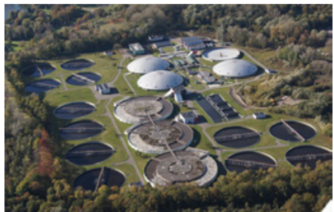
Figure 3.5 A typical activated-sludge WWTP, in this case the WWTP of Eindhoven (Photo retrieved from www.duurzaamvastgoed.com )
