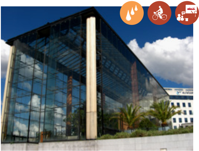
Figure 4.2 Design criteria: a decentralized WWTP that is integrated in its spatial context (1). This is an example of how the WWTP could look like in its urban context ( www.patryst.com )
