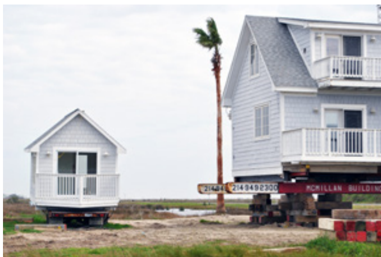
Fig 9: Lifting of houses for flood-proofing
