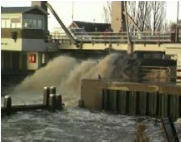
Figure 3.4.7 | Temporary increased pumping capacity in Zwartsluis during the 1998 flooding.
