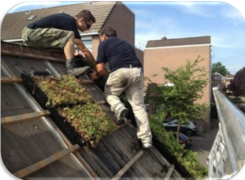
Installation of the Ecopan ( www.pioneering.nl ).
