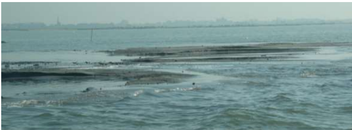
Sand nourishment of Workumer Buitenwaarden a pilot project just after construction in 2011 (source: https://publicwiki.deltares.nl/ ).
