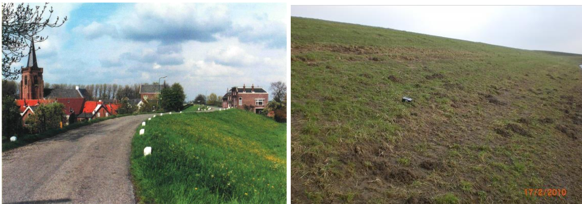
Figure 1.5 Left: a typical Dutch grass dike, right: damage to a Dutch dike due to tire tracks (source: Digigids)
