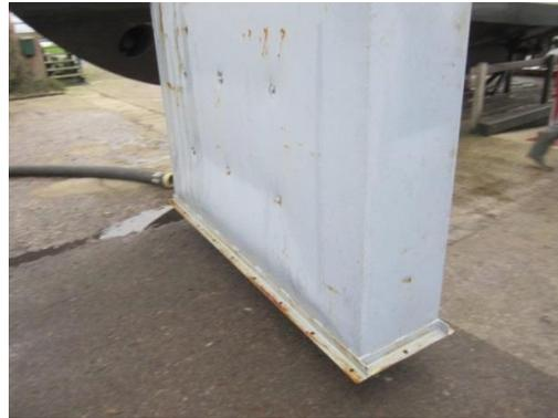
Picture 35. Bended lower module water column
