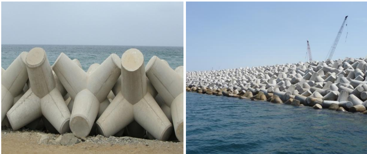
Figure 1.4 Crablock armour units as monolayer system in breakwaters at Al Fujeirah [Source: Hendrikse (2014)]
