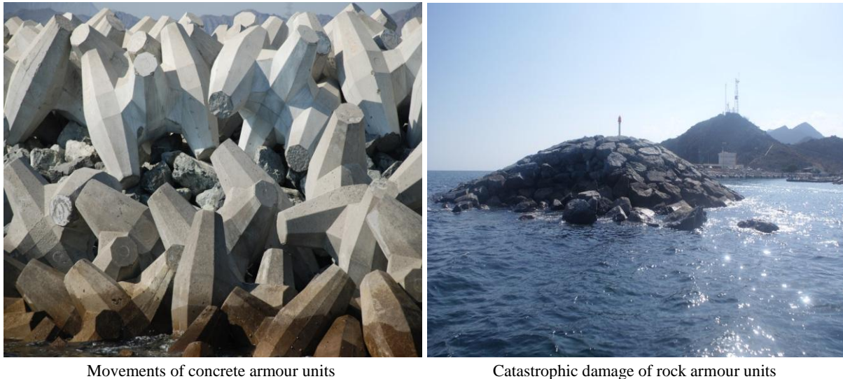
Figure 1.2 Consequences of cyclone on breakwaters in Al Fujeirah [Source:Hendrikse (2014)]
