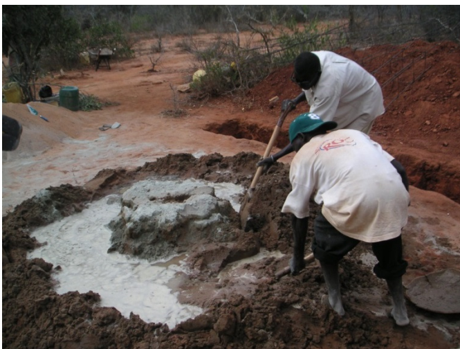
Figure 20 Mixing the mortar
