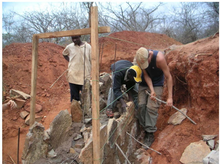
Figure 19 Casing of the dam without wood but by using flat stones
