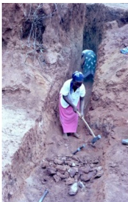
Figure 16 Digging with a hammer and chisel
