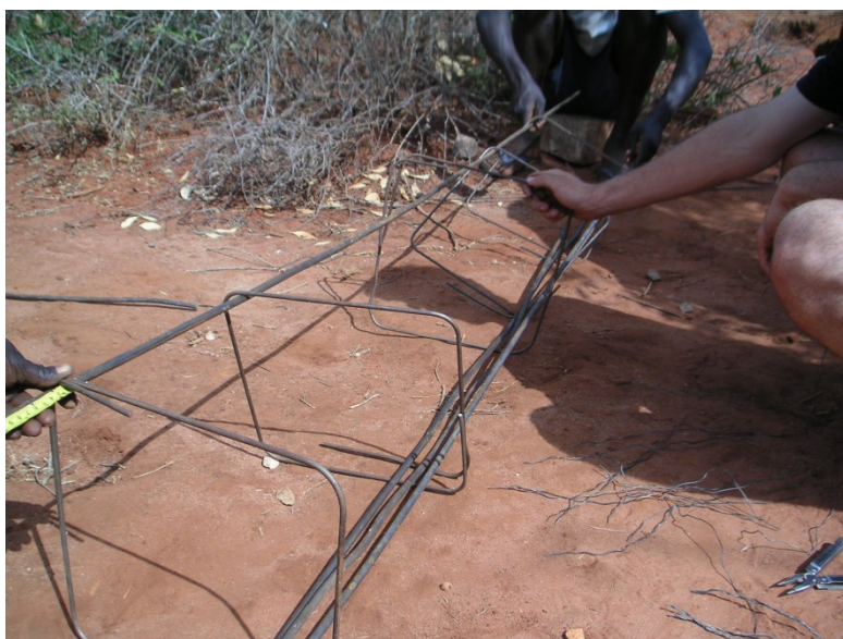
Figure 18 Constructing the reinforcements for the concrete
