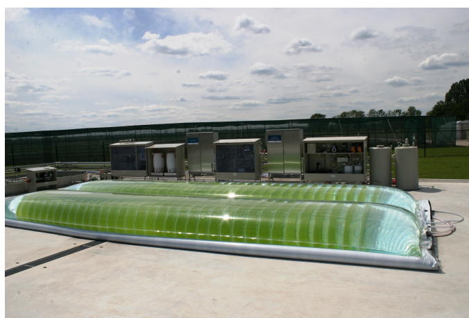
Figure 2-6: Flat panel PBR at AlgaePARC (Netherlands)
