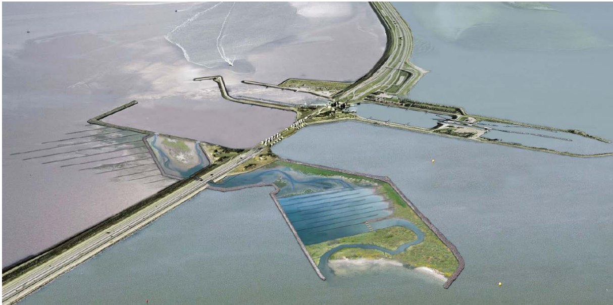
Figure 6 Impression of the fish migration river at the Afsluitdijk, enabling the formation of saltmarsh at the Wadden Sea side of the dike. Source: http://www.deafsluitdijk.nl/wp-content/uploads/2014/11/InteractievePDFVismigratierivierDEF.pdf
