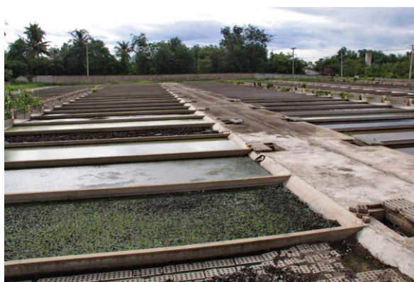
Figure 23. Air-drying of bioslurry on shallow plateaus on a large pig farm in Thailand.
