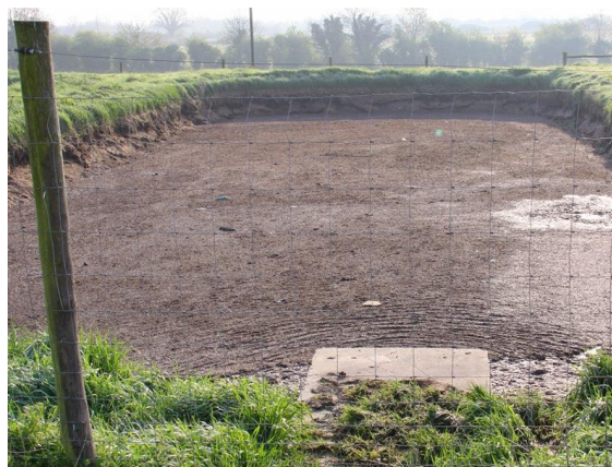
Figure 18. Cattle slurry stored in an uncovered lagoon.
