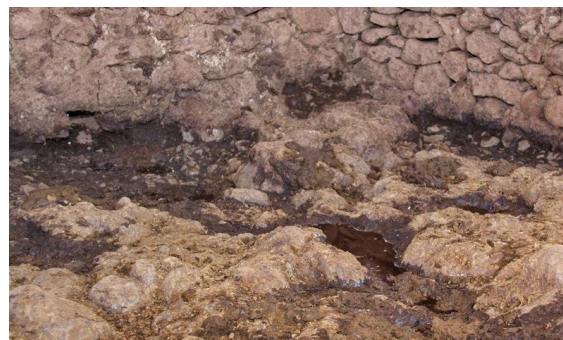
Figure 12. Bad flooring makes it hard to collect dung and urine, and is very uncomfortable for cattle to stand or lie on.
