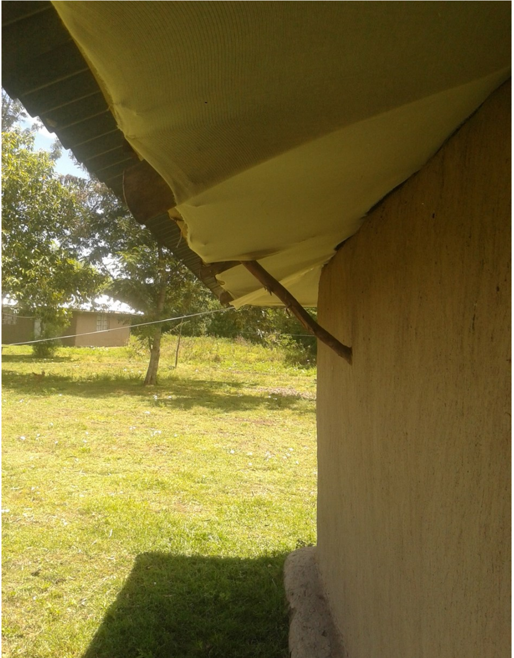
Supplementary Figure 2. Eave screening with cotton net fabric, experiment II. The fabric was fixed using a staple gun, and rather than applying it to cover only the eave it was stapled to the wooden beam that forms the top of the wall and then stretched outwards and fixed on the outermost wooden beam which supports the roof.
