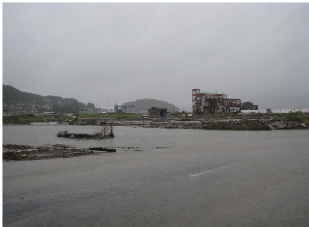
Figure 26: Left: Subsided land near the shoreline; Right: Evacuation building on the waterfront that was just overtopped, people sheltered on the top of it survived (The 2011 Tohoku Earthquake Tsunami Joint Survey Group; www.coastal.jp/tsunami2011 )
