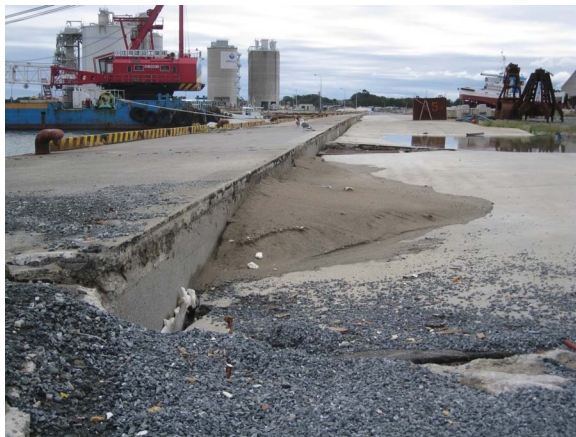
Figure 46: Subsidence of quay wall and under-flown liquefied sand
