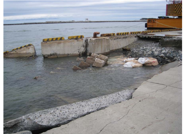
Figure 45: Damage of quay wall and fallen apart post-tsunami retaining measures
