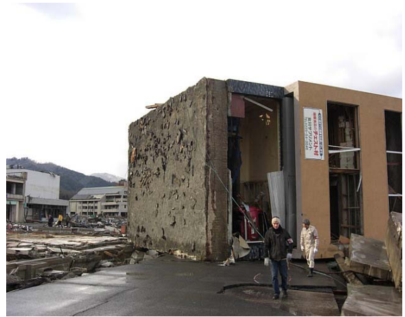
Figure 31: Overturned buildings (Left: The 2011 Tohoku Earthquake Tsunami Joint Survey Group; www.coastal.jp/tsunami2011 )
