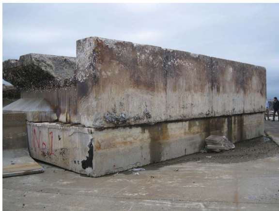
Figure 47: Overturned quay wall elements
