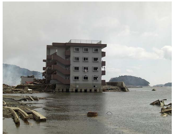
Figure 26: Left: Subsided land near the shoreline; Right: Evacuation building on the waterfront that was just overtopped, people sheltered on the top of it survived (The 2011 Tohoku Earthquake Tsunami Joint Survey Group; www.coastal.jp/tsunami2011 )
