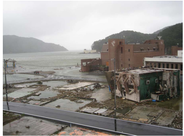
Figure 30: Devastated waterfront of Onagawa. Note the overturned building on the right picture.
