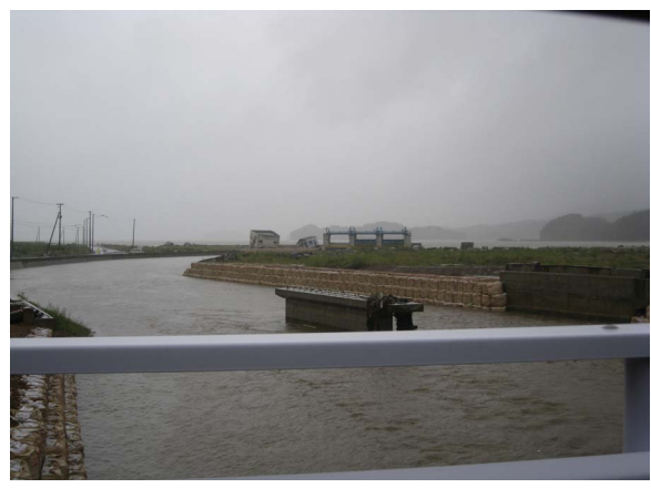
Figure 27: Left: Severely damaged storm-surge gates (The 2011 Tohoku Earthquake Tsunami Joint Survey Group; www.coastal.jp/tsunami2011 ) Right: Temporary retaining measures on the riverbanks and lone standing bridge abutments. The slab was washed away.
