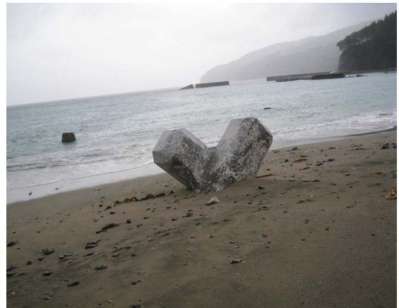
Figure 11: Left: Detached tsunami gate; Right: Severely damaged caisson breakwater. The armour unit was part of its outer side protection.
