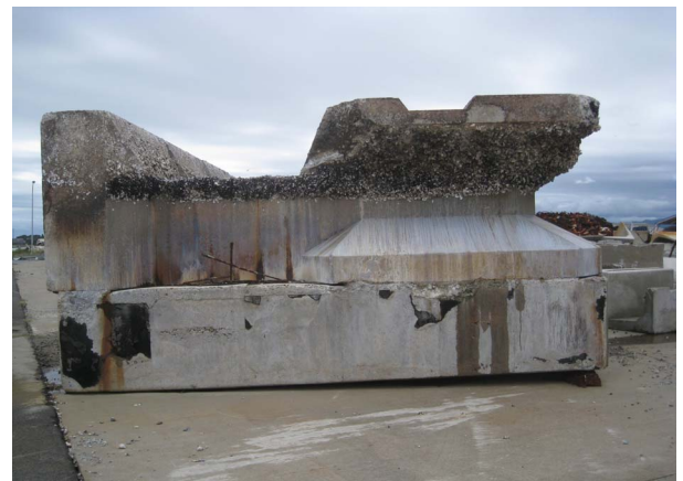
Figure 47: Overturned quay wall elements
