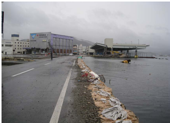
Figure 21: Left: Temporary land protection, Right: Destroyed warehouse on former quay wall
