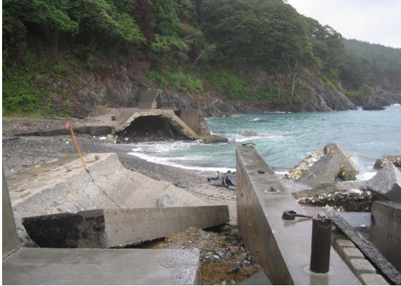
Figure 10: Left: Large breakage of tsunami wall in Ryori; Right: Temporary protection measures against storm surges.
