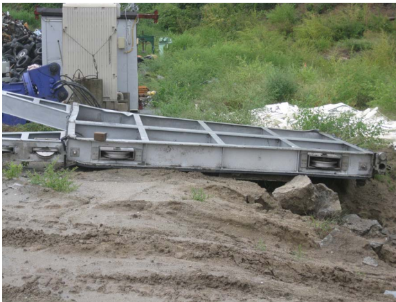
Figure 11: Left: Detached tsunami gate; Right: Severely damaged caisson breakwater. The armour unit was part of its outer side protection.
