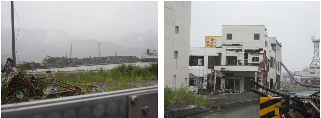
Figure 7: Left: Accumulations of debris in Ofunato port; Right: Damage of steel frame building. The height of the damage is indicative of the inundation height.
