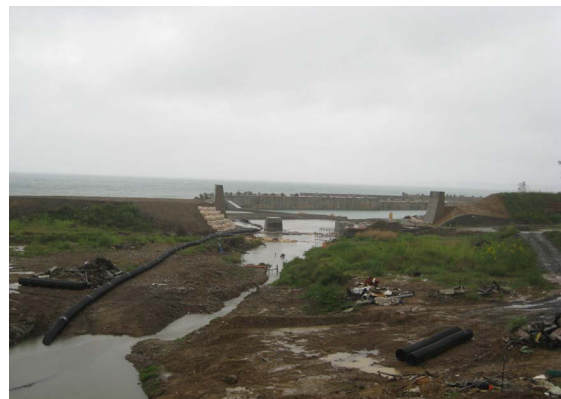
Figure 22: Left: Subsided land, Right: Retaining works at severely subsided land near Kesennuma
