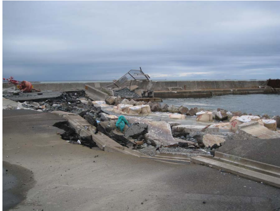
Figure 45: Damage of quay wall and fallen apart post-tsunami retaining measures
