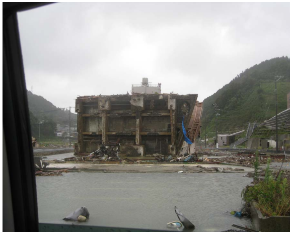
Figure 31: Overturned buildings (Left: The 2011 Tohoku Earthquake Tsunami Joint Survey Group; www.coastal.jp/tsunami2011 )
