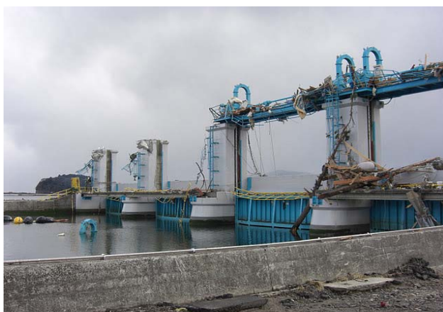
Figure 27: Left: Severely damaged storm-surge gates (The 2011 Tohoku Earthquake Tsunami Joint Survey Group; www.coastal.jp/tsunami2011 ) Right: Temporary retaining measures on the riverbanks and lone standing bridge abutments. The slab was washed away.
