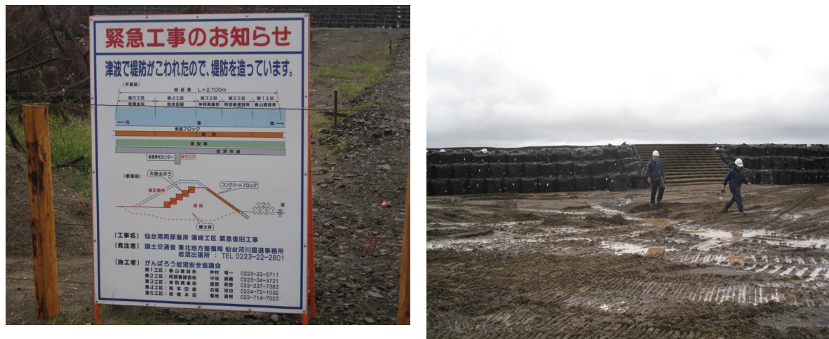
Figure 41: Left: Plan for temporary retaining works, indicated with orange. The original cross section is indicated with grey; Right: Sandbags placed urgently the day of the visit (September 22, 2011), as the cross section was further destroyed by typhoon Roke.
