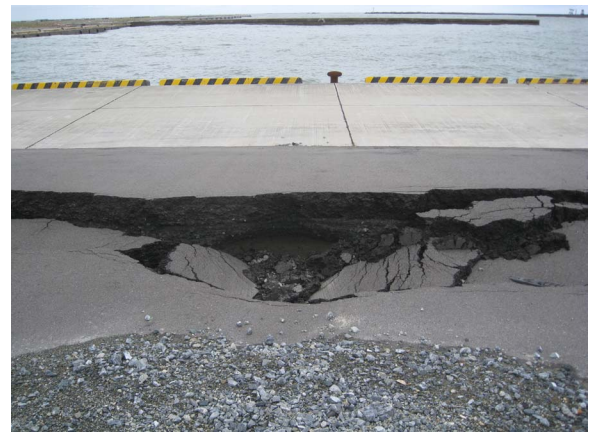
Figure 46: Subsidence of quay wall and under-flown liquefied sand
