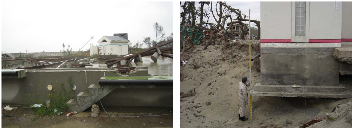
Figure 34: Left: Devastated buildings behind the dike, Right: Scouring on the toe of concrete building (The 2011 Tohoku Earthquake Tsunami Joint Survey Group; www.coastal.jp/tsunami2011 )
