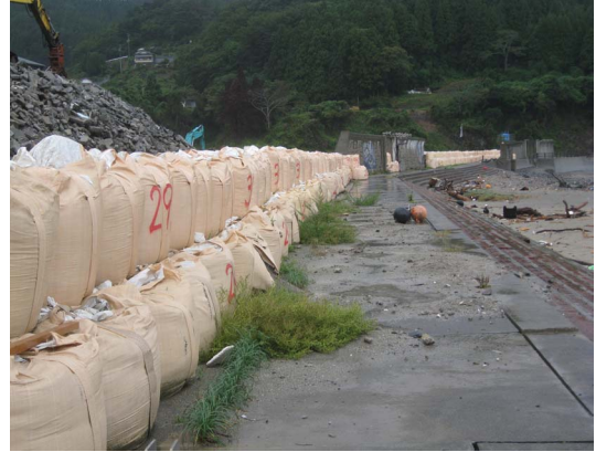
Figure 10: Left: Large breakage of tsunami wall in Ryori; Right: Temporary protection measures against storm surges.
