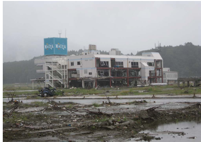
Figure 15: Left: Concrete building that survived. It might have also been evacuation building. Right: Damage on steel frame building.
