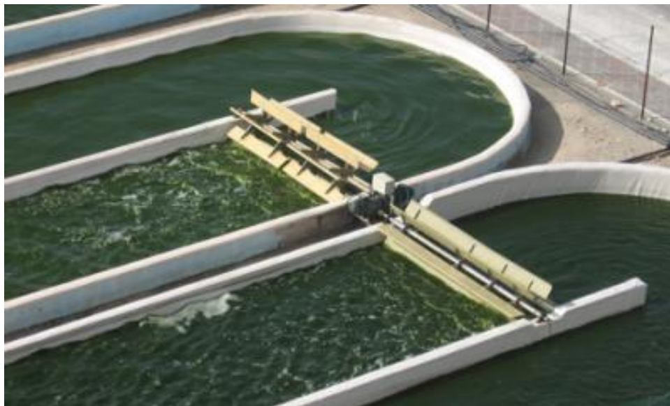
Figure 13: High Rate Algal Ponds (HRAPs) (ECN, 2014).
