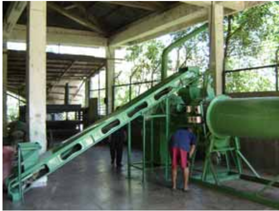
Figure 36 The covered transportation belt
