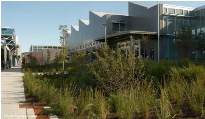
Photo 1 Kensington High School manages all stormwater on site using green roofs, rain gardens and more. (Focht 2013)
