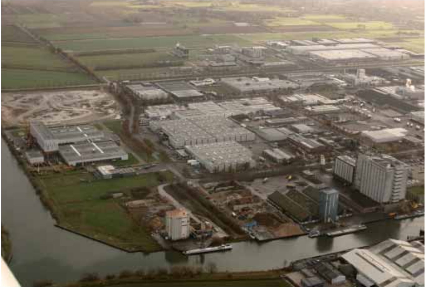
Industrieterrein Elzenburg te Oss.
