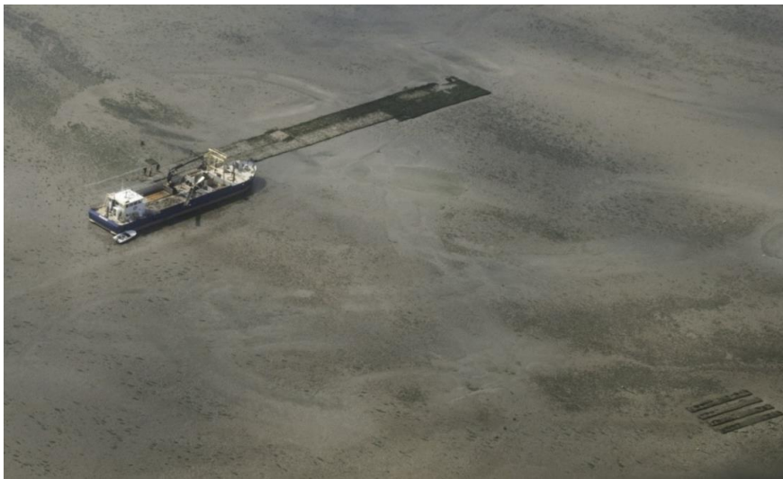
Figure 1.5 Aerial photograph of the intertidal artificial oyster reefs in the Oosterschelde estuary. Picture was taken during the construction of one of the large artificial oyster reefs (VianeWest) in 2010. In the right corner, one of the small Pilot reefs constructed in the summer of 2009 is visible. Photo credits: L. Adriaanse
