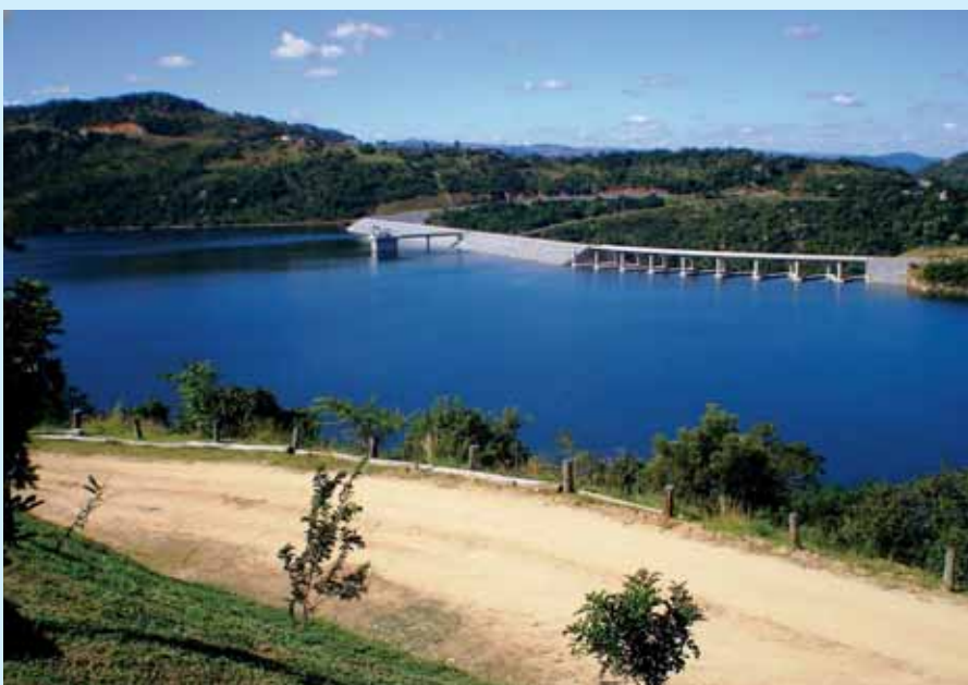
De Maguda-dam (foto: Warry Meuleman).
