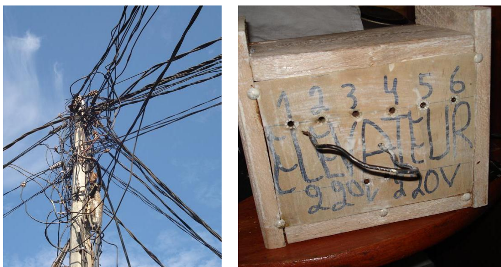
Figure 3.2: DRC – cable network and self-made device to raise the voltage (pictures taken by Nynke Douma)
