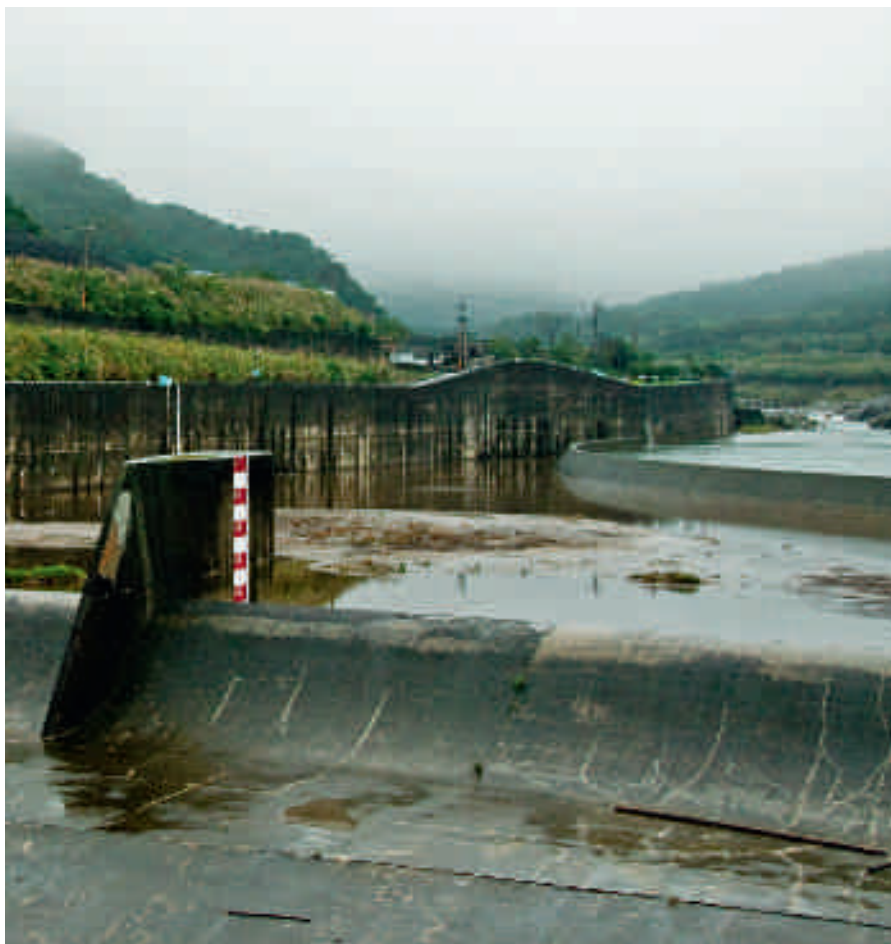
De Yuanshantze Flood Diversion Tunnel.
