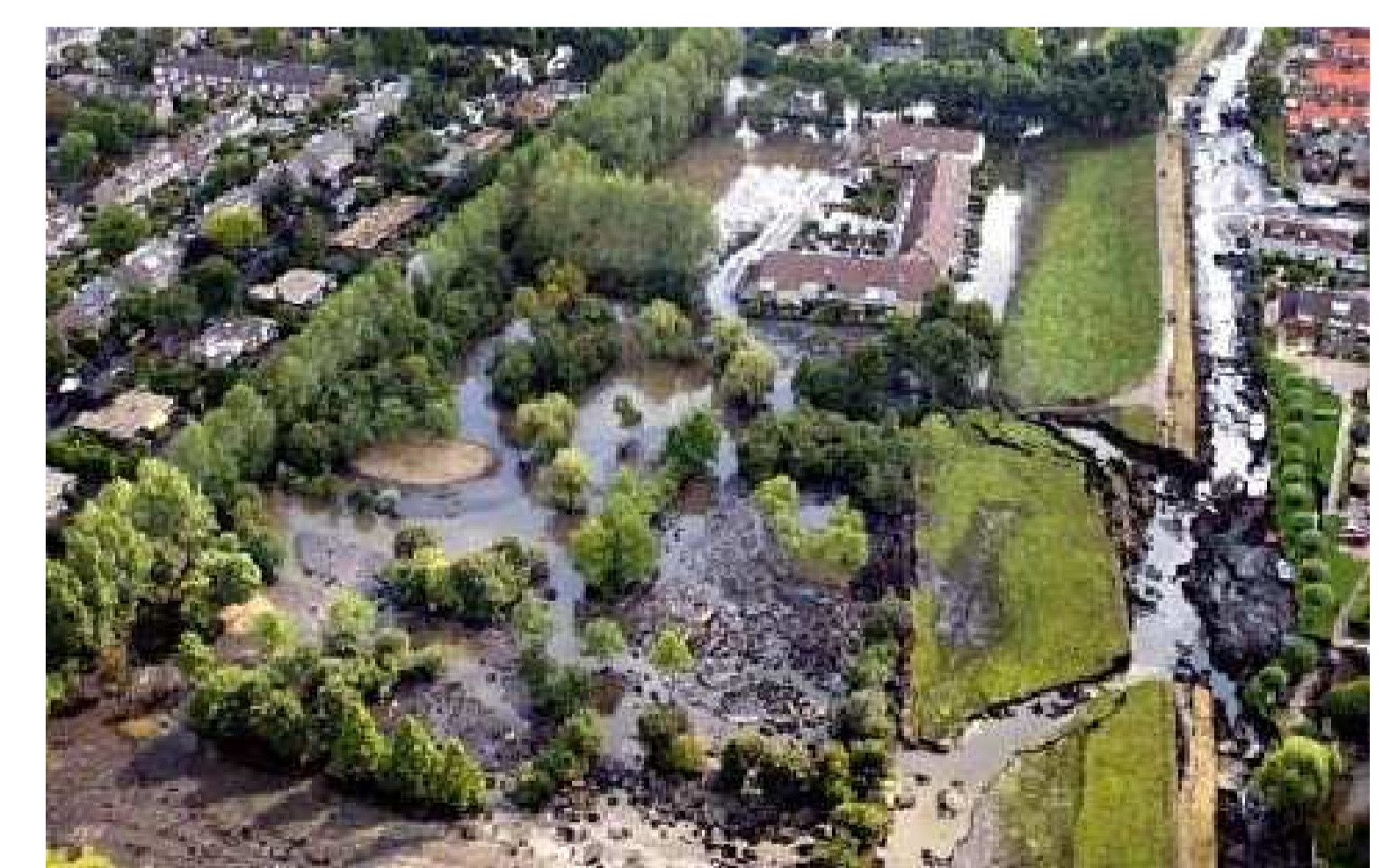
Figure 6: Dike failure.
