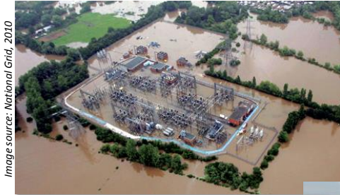
Flood vulnerability of electrical substations
