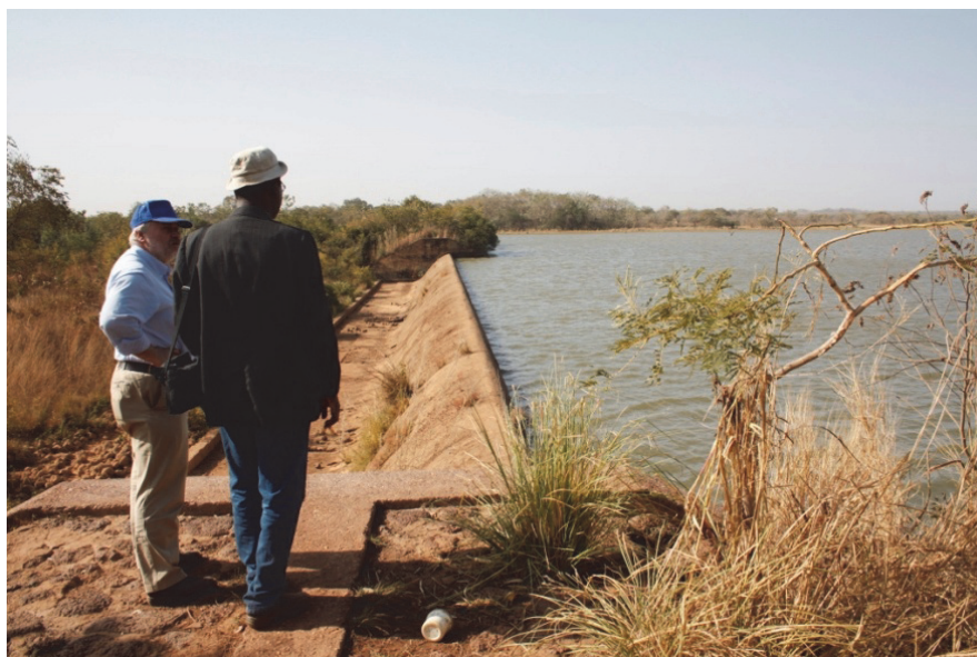
Figure 3.4: Spillway of Tiefora earthen dam
