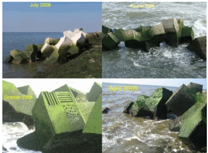
Xbloccs covered with algae - IJmuiden. Bron: http://www.xbloc.com/
