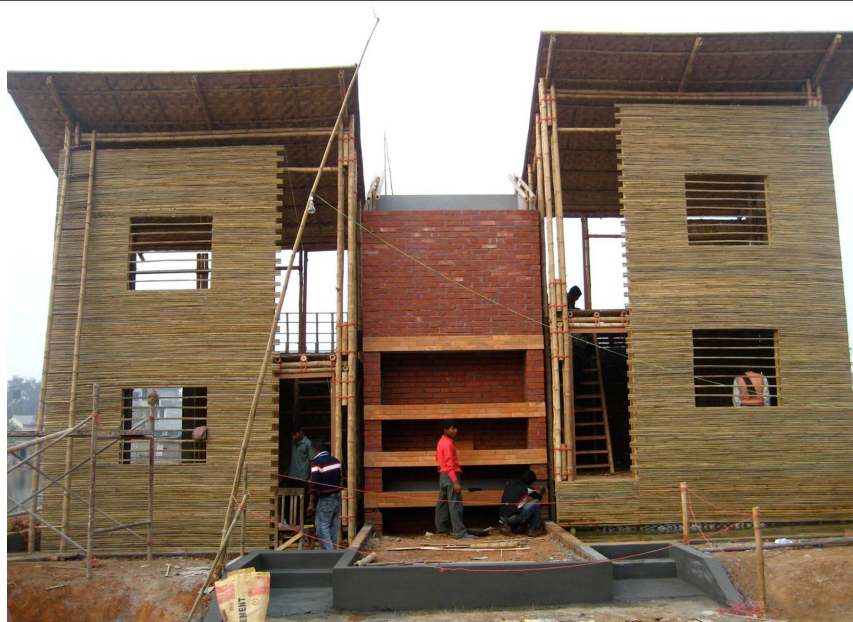
Day 66 – "You will notice in Photo25...the house on the right is higher than the left.. its floating!" (this has the recapped plastic bottle buoyancy blocks)
