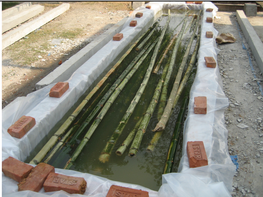
Day 15 – Bamboo poles are submerged in chemical for treatment
