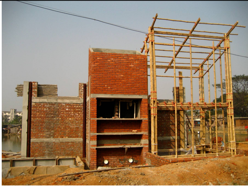
Day 46 – Brick work is finished and bamboo frame for one dwelling is started
