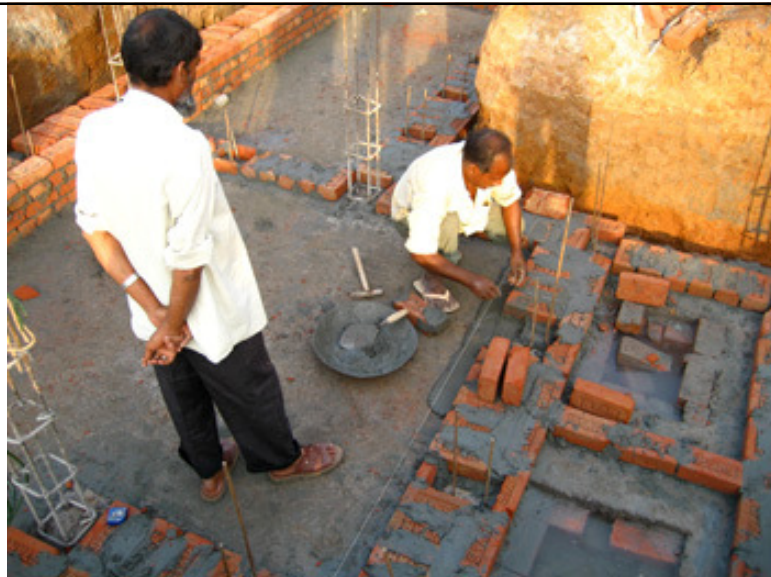
Starting the brick walls for the composting latrines and rainwater storage cisterns
