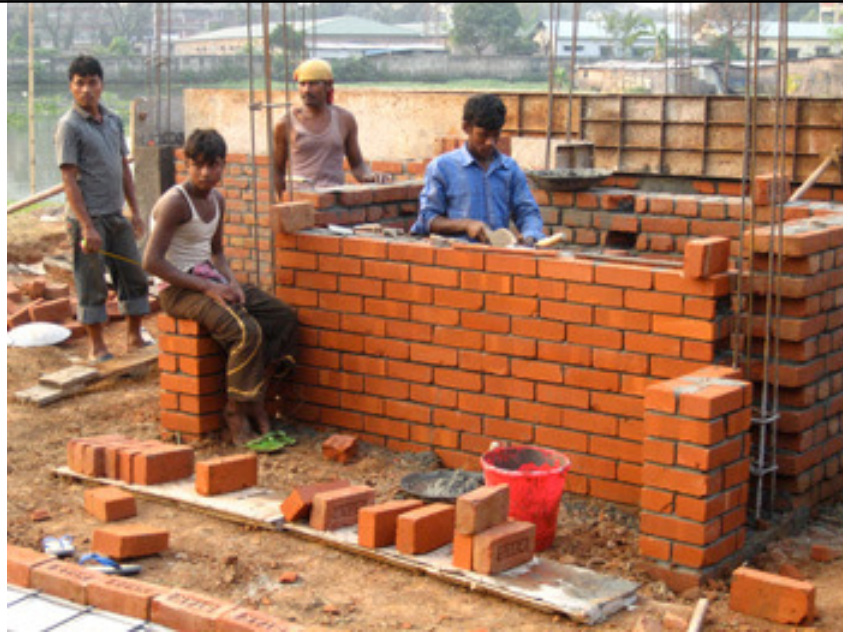
Building up the water storage cistern walls
