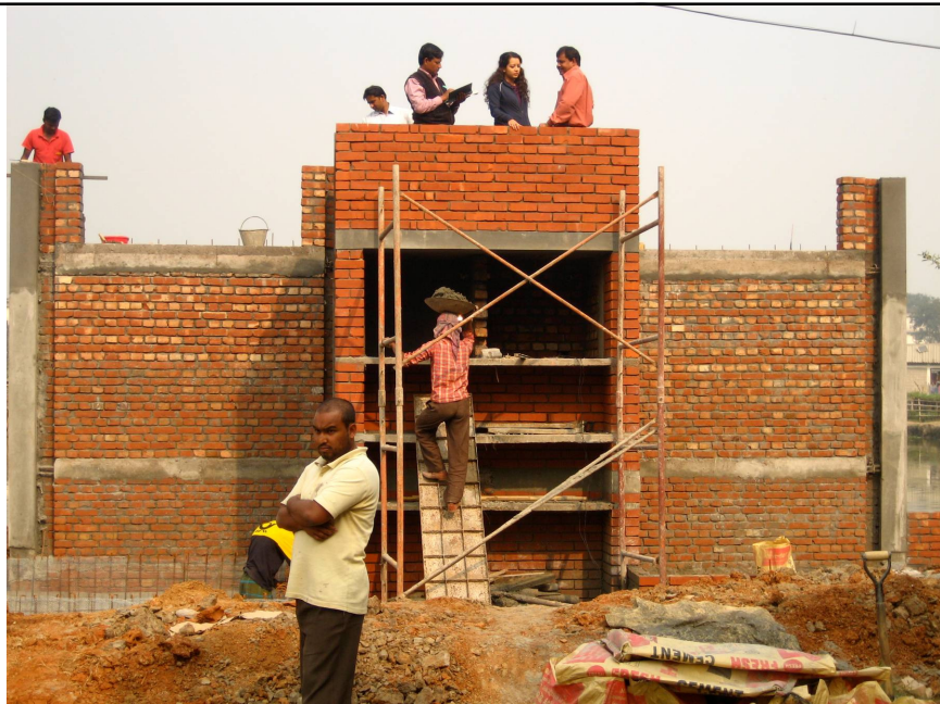
Day 32 – water cistern top slab and brick walls with concrete beams are finished
