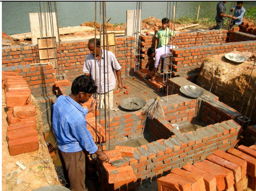
Day 10 – Brick foundation walls are started for water cisterns and composting latrine storage
