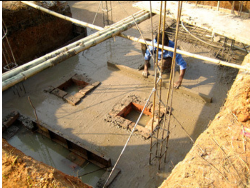
Concrete foundation for the service core
