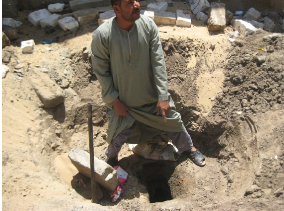
1. A not functioning infiltration tank.
