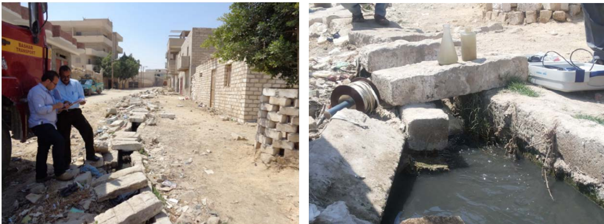
Photo 9 Left: Main collecting sewer (mostly for grey water and black water is partially mixed). It is excavated and built with limestone bricks, covered and extends along main road of the village, it drains by gravity into lake, waterfall and wetland. Right: Main collecting sewer before discharge into lake.
