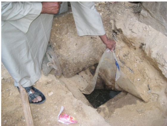
3. A not functioning infiltration in the low clayey area
