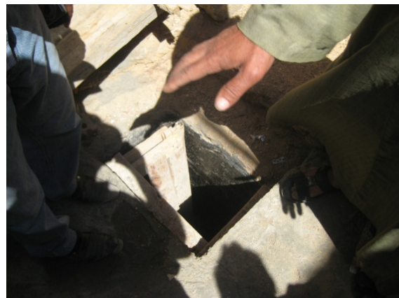
2. A well-functioning infiltration tank in the higher sandy area
