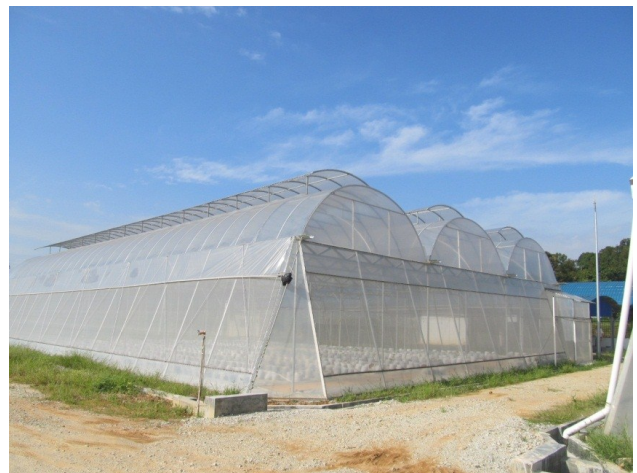
Greenhouse realized in Malaysia, suitable for a tropical climate. The greenhouse has a 2-sided top opening, tilted sides, nets along the sides that allow air entrance. With a mature, fully transpiring crop, an indoor temperature below the outdoor temperature is realized (Elings et al., 2012).
