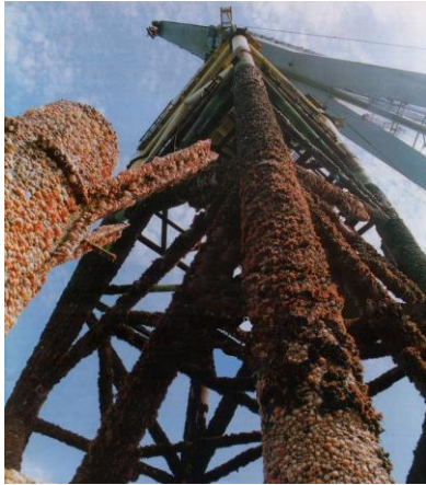
Figure 5-1. Biofouling on an offshore jacket foundation.
